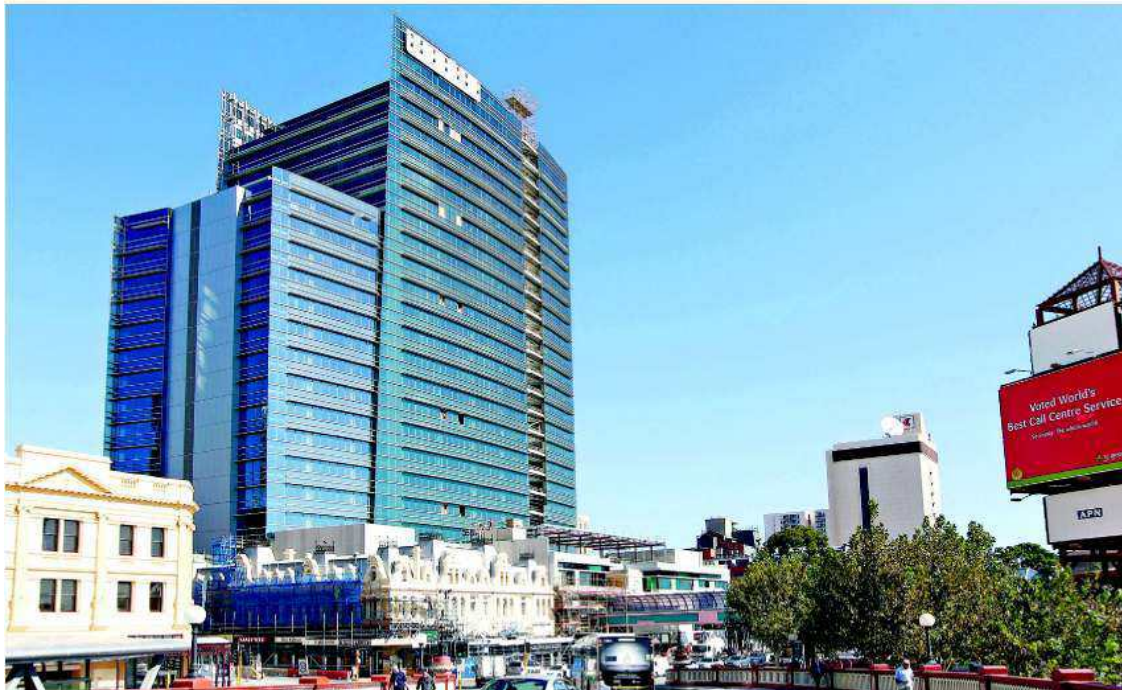
Finishing off: Probuild is finishing off the Raine Square building after a dispute ended the contract of the original contractor.
